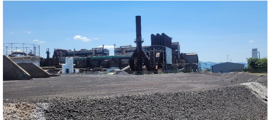
Smelter Plant, currently non-operational.
