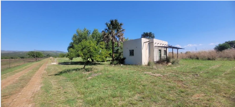
Existing building structures.
