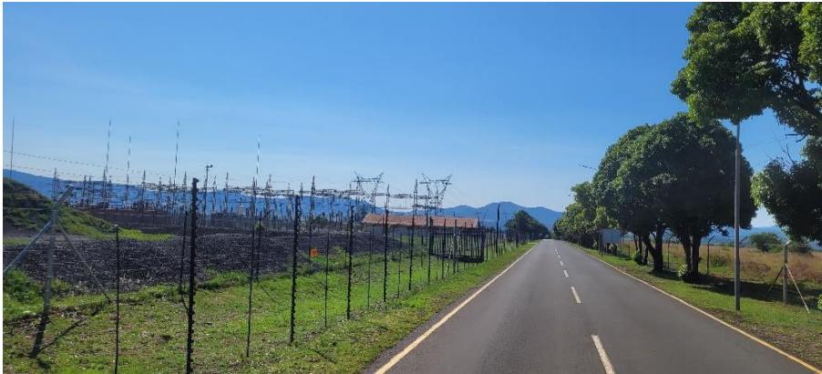
Main access road and existing services including Eskom Substation.
