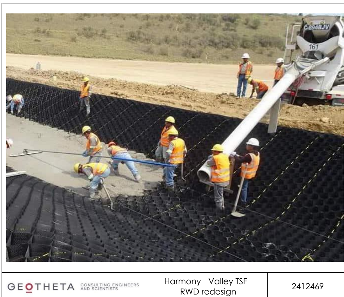
Figure 17: Construction of concrete filled HDPE geocells
