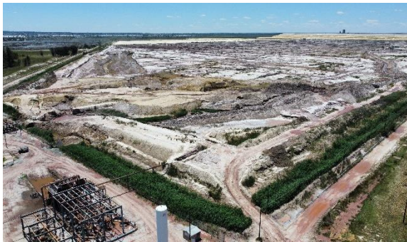
Figure 17: Aerial view of the Brand A TSF (active reclamation underway)
