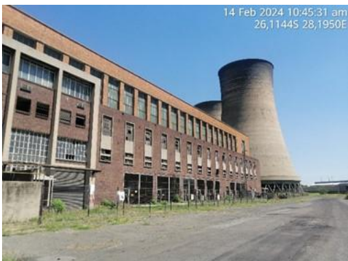
Figure 11: View of the Kelvin A-station, cooling towers and access road
