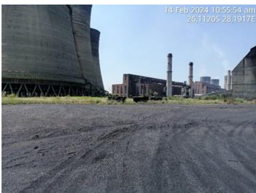
Figure 13: General conditions of the study area.
