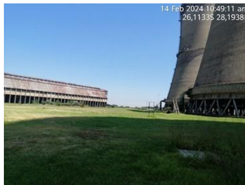
Figure 12: Kelvin A-station cooling towers (CCGT Power Plant footprint)
