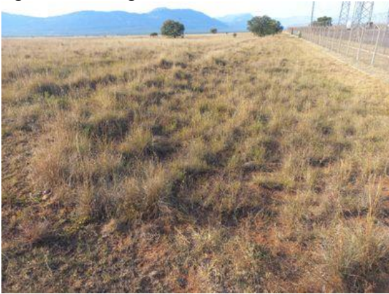
Figure 21: View of cut from which Delphi Substation was levelled.
