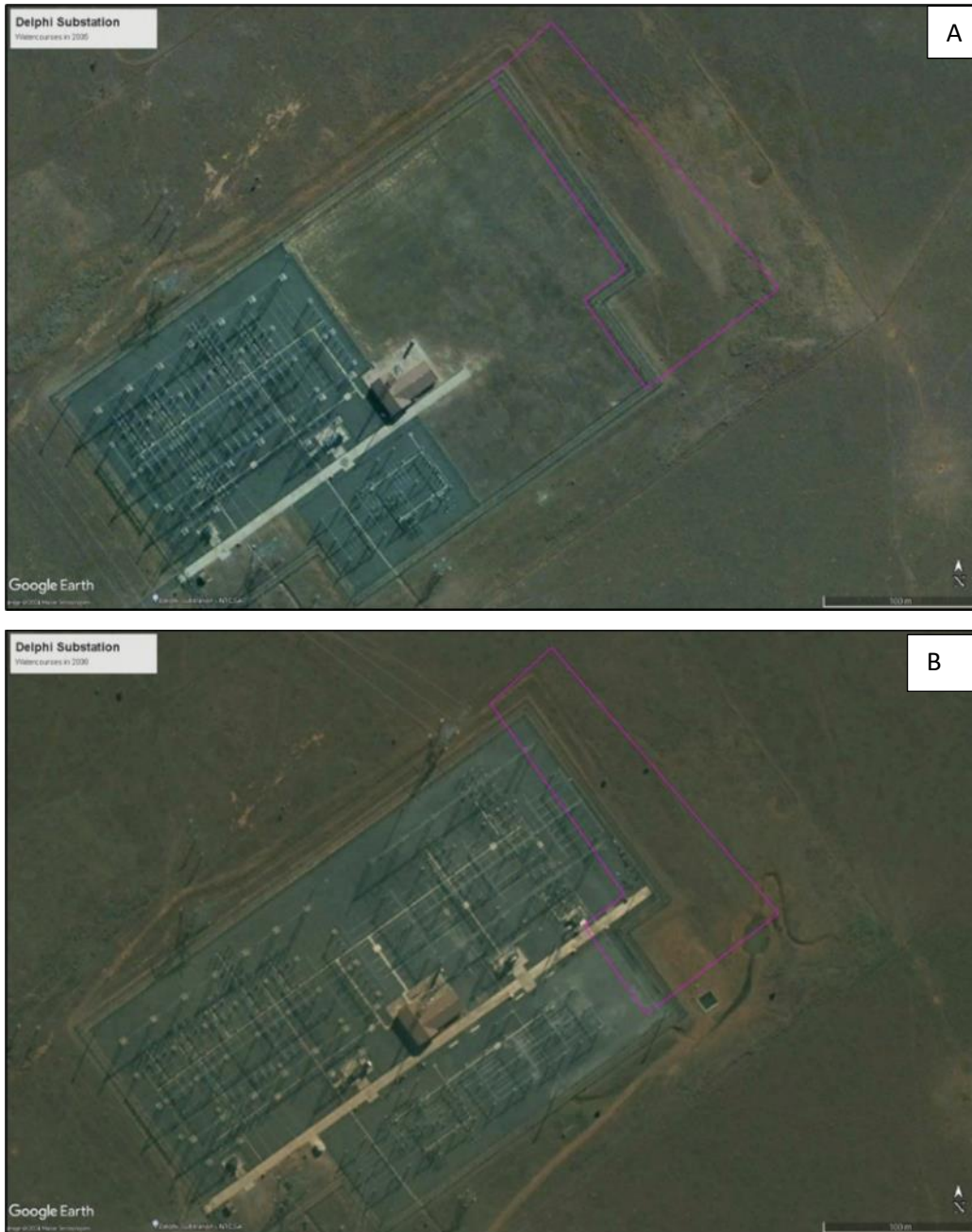
Figure 18: Delphi Substation Google Earth Image 2005 (A) and Delphi Substation Google Earth Image 2008 (B)
