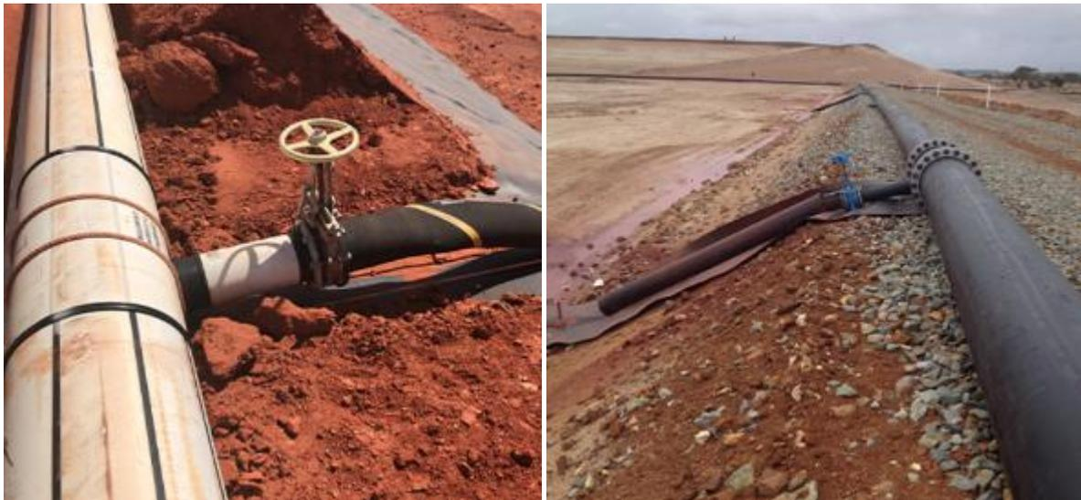
Figure 42: Example of spigot deposition. Spigot at a pre-constructed embankment crest (left) and spigot pipes laid along the main wall (right) (Goldfields, 2023).
