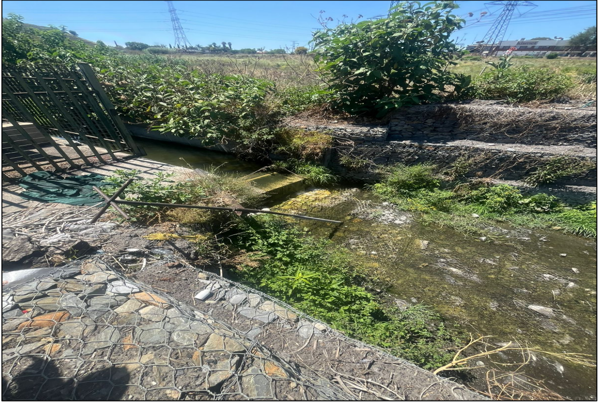
Photo site 5: Showing downstream point to Modderfontein Spruit river.
