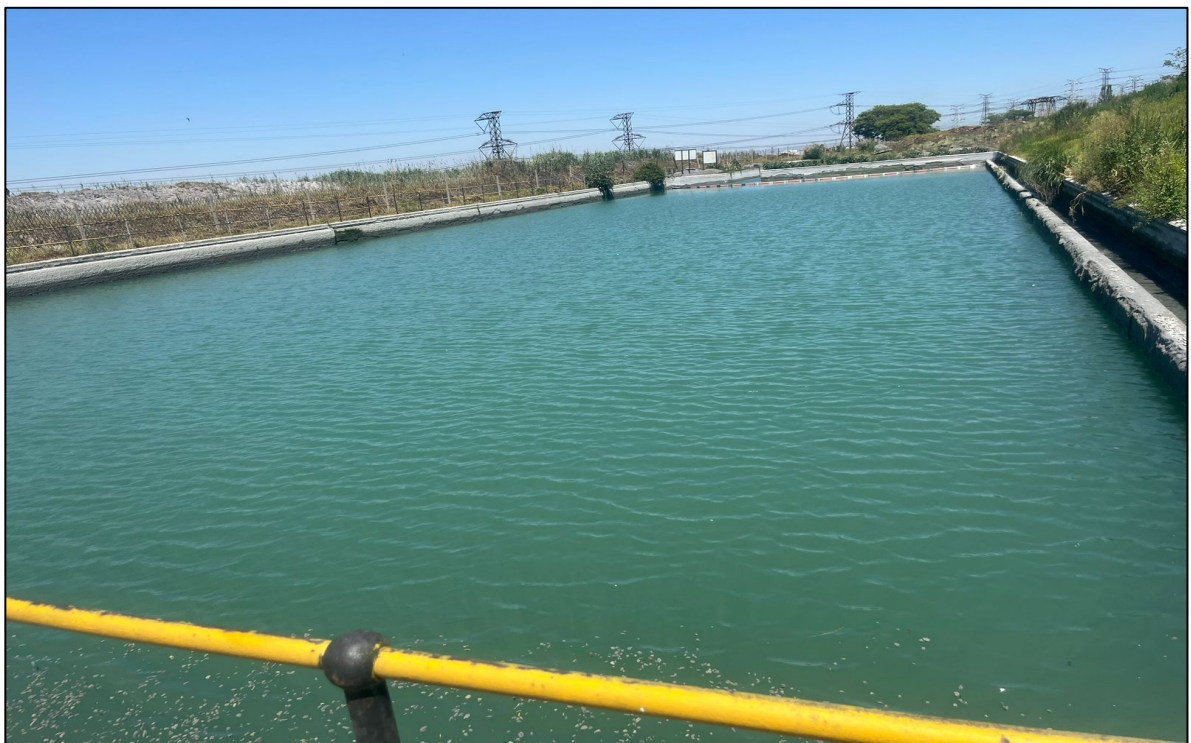
Site Photo 4: Showing the return dam
