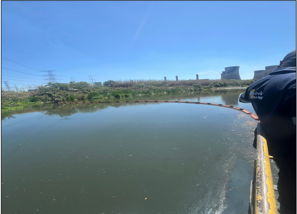
Site photo 3: Showing de-silting dam
