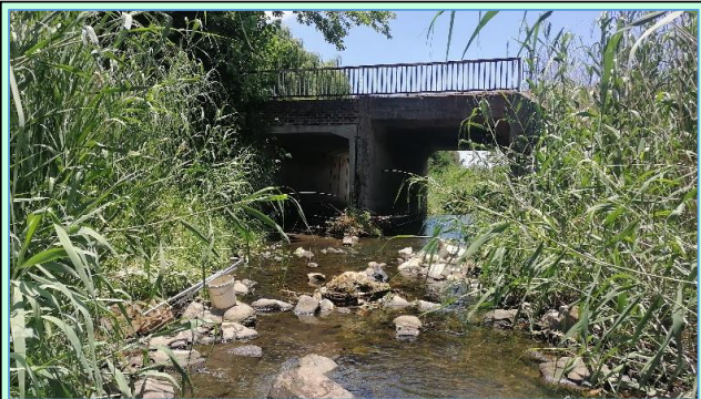
Plate 6: Downstream view of site K2 (2024-11)
