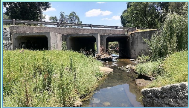
Plate 2: Downstream view of site K1 (2024-11)
