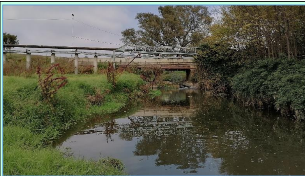
Plate 16: Upstream view of site K4 (2024-05)
