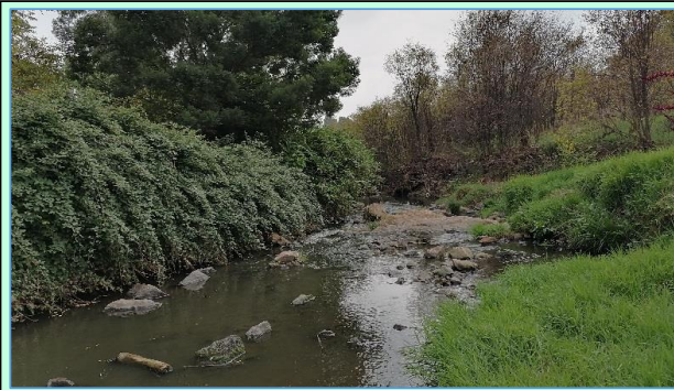
Plate 17: Downstream view of site K4 (2024-05)
