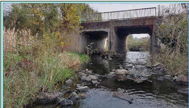
Plate 8: Downstream view of site K2 (2024-05)
