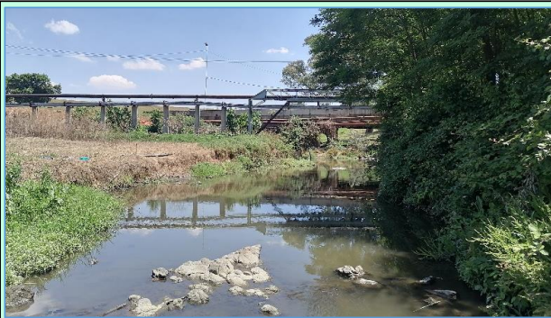
Plate 14: Upstream view of site K4 (2024-11)
