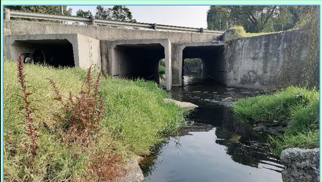
Plate 4: Downstream view of site K1 (2024-05)
