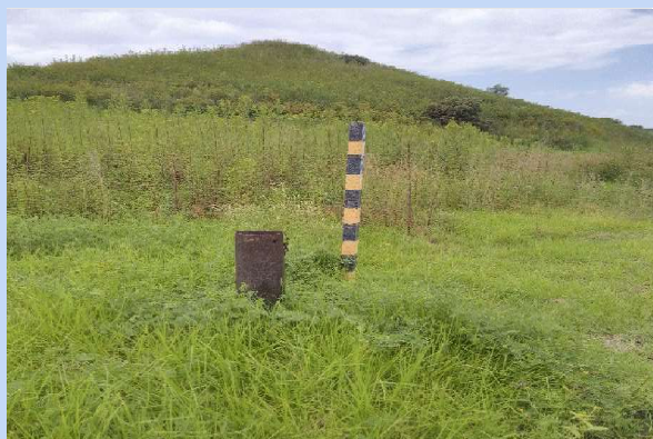
Borehole on Western Perimeter - Toe of Ash Dam B
