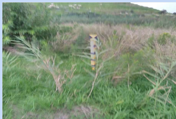
Borehole on Southern Toe of Ash Dam B
