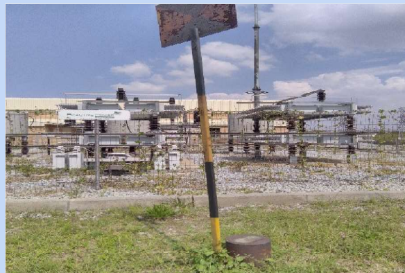
Borehole North of Ash Dump - North Western Perimeter
