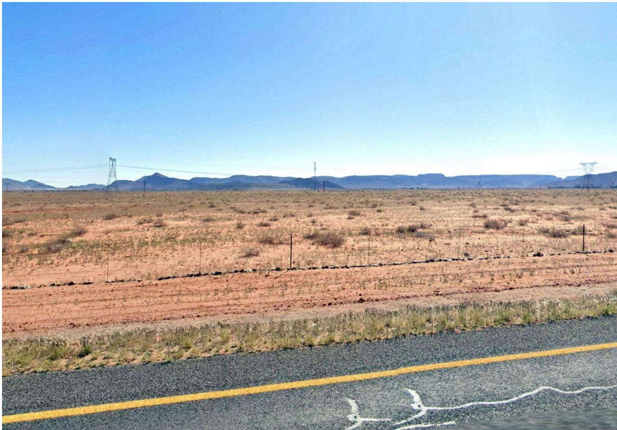
Figure 39: A 400kV overhead powerline running parallel and approximately 250m from the N14 close to the Aggeneis Substation.
