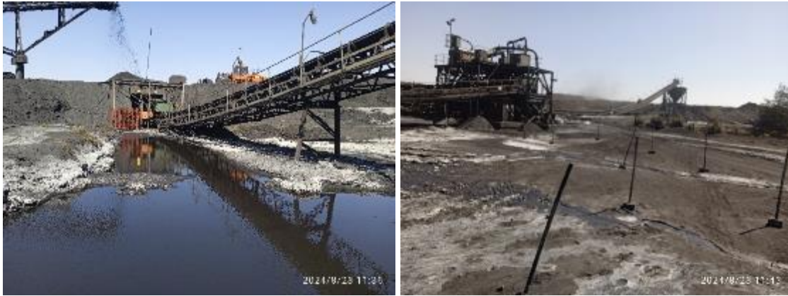
Figure 9: Potentially contaminated run-off water from the wash plant by passing the silted PCD and flows to the wetland.
