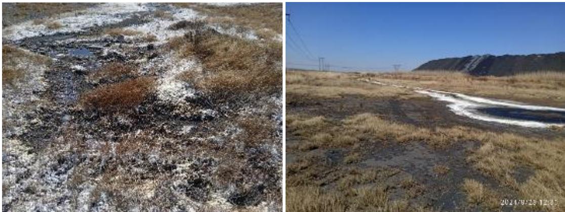
Figure 22: Visual observation traces of seepage potentially from the co-disposal facility on the northern-western side of the facility. This has potential to impact the Witpuntspruit from upstream (WT-S01) to downstream (WT-S06) if no interception is undertaken.
