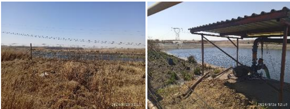
Figure 14: Co-disposal Dam 3 and Dam 1.
