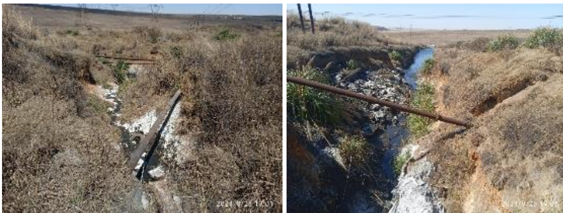
Figure 17: Erosion of the channel discharging potentially contaminated stormwater into the wetland on the north-eastern side.
