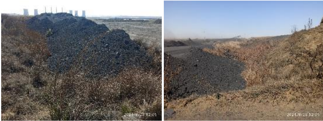
Figure 18: Discarding of potentially contaminated material onto the stormwater channel along the RoM.
