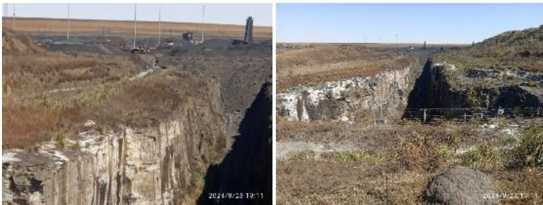
Figure 13: Underground operations ceased end of 2021 and back filling has commenced as part of rehabilitation.
