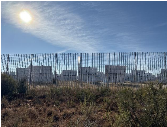
Figure 23: Outer CSP fence separating the study area from the existing CSP.
